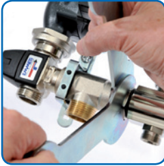
Fig. 5 Tightening the swivel joints
